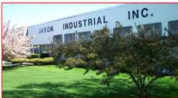
Sede Corporativa Jason Industrial Fairfield, NJ
